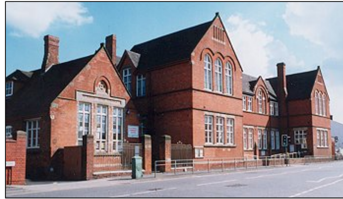
Blakenhall Community Centre, Dudley Road.
